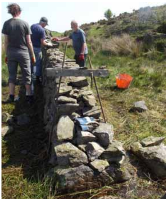
Plate 5: Properly aligned faces, and a good heart – the wall takes shape
