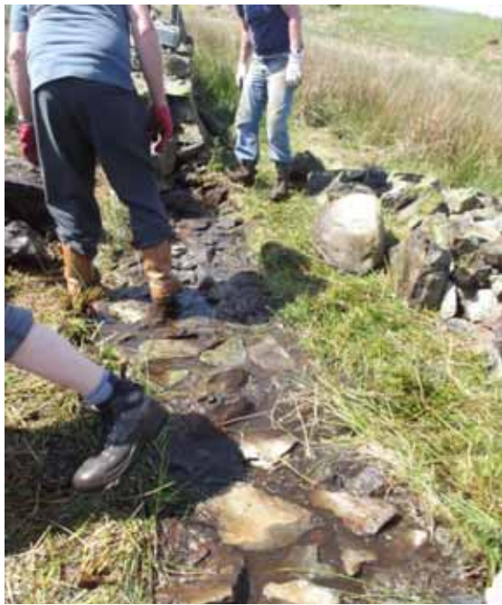
Plate 3: Any new build structure requires a reasonable foundation
