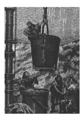
This nineteenth Century print records the sinking of a shaft at the point just below "rock head" where conditions are suitable for the excavation not to require support. In this case the shaft is brick lined, and would most probably have been sunk as a caisson. This involves simultaneous laying of brickwork, and cutting away the toe so that the lined shaft sinks under its own weight, until it reaches an appropriate footing.
